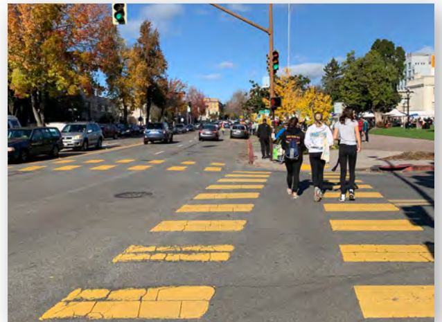
Martin Luther King Jr. Way at Allston Way. Crossing pedestrians and left-turning vehicles are in conflict.
