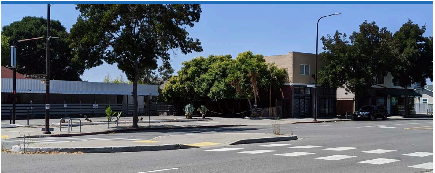
This pedestrian crossing at Sacramento Street and 66th Street includes a median refuge island, allowing pedestrians to cross two lanes of traffic at a time.
