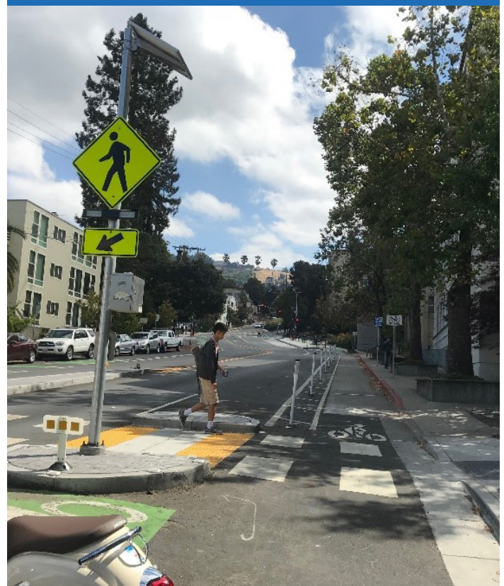
A pedestrian crosses Hearst Avenue at a marked crosswalk. This crossing has a rapid flashing beacon and a median island. Photo: Amanda Leahy, Kittelson
